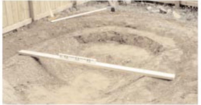
Leveling the pond during construction.
